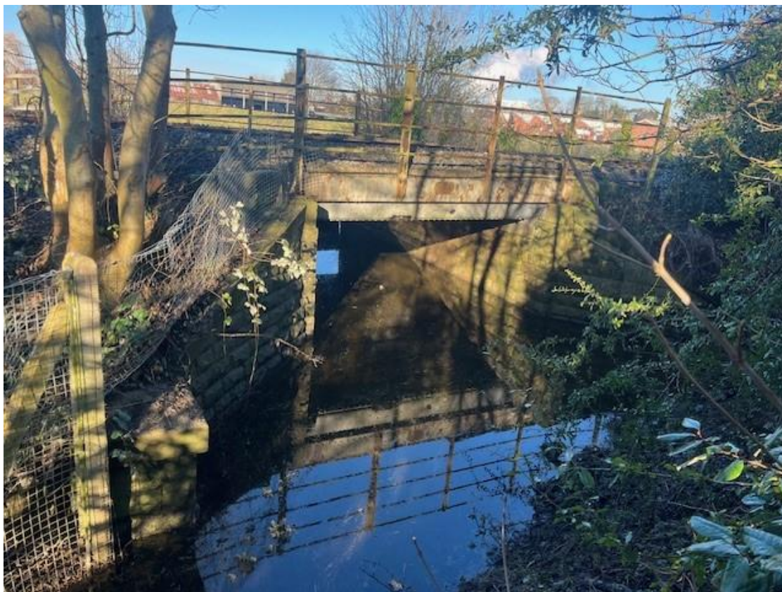
Figure 14: Photo of the existing culvert to east and the associated ditch or trackway. Source: Skanska, 16/01/2025.
